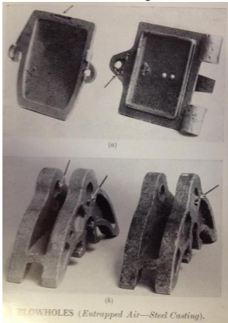
Both of the pictures (a) and (b) are small castings with wall thicknesses ranging from 6 – 19mm in cross section. Both items were cast in green sand.
